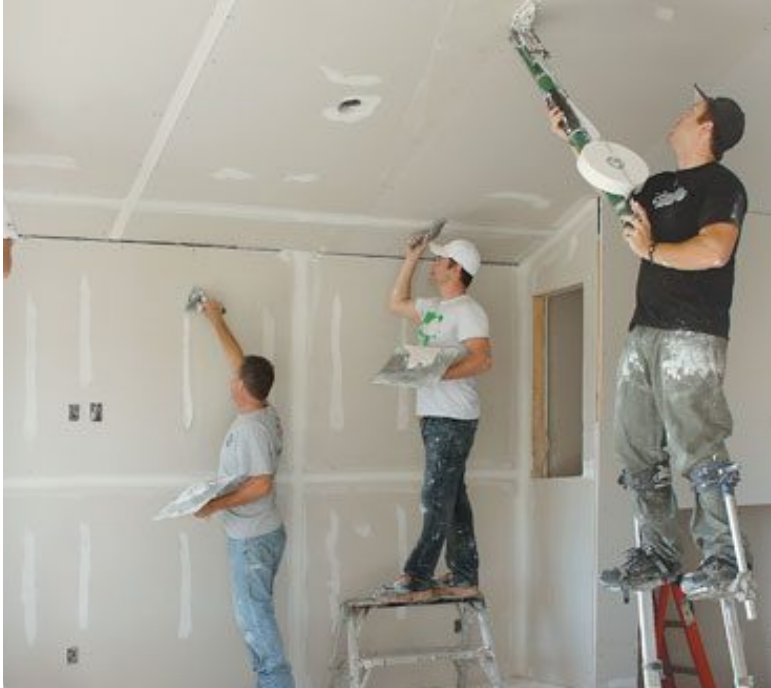
SERVICE 04 / DRYWALL FINISHING
